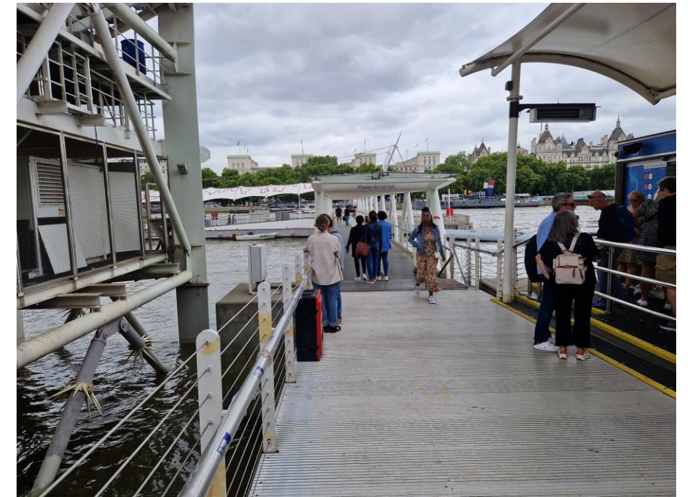
Transfer to the pontoon from the ticket office
